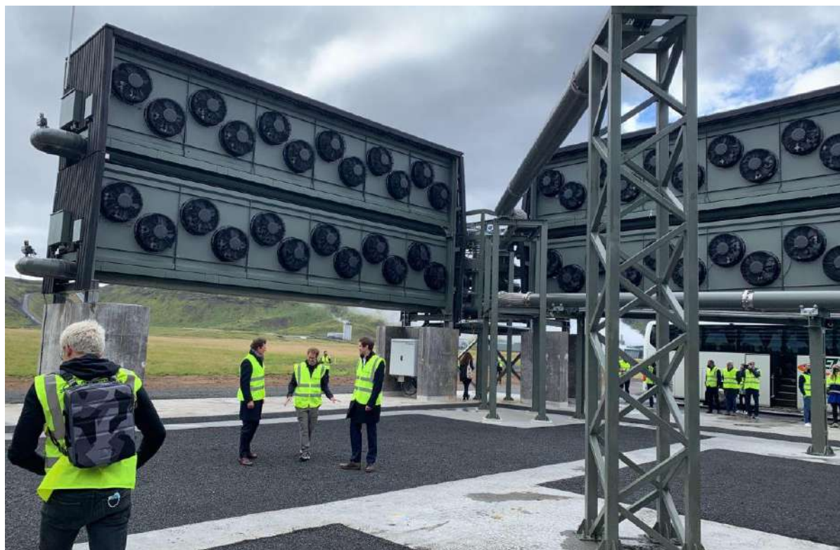
Innovative materials are important for enabling point-source carbon capture systems and CO 2 removal systems, such as this direct air capture (DAC) plant in Iceland (photo credit: Julio Friedmann).
